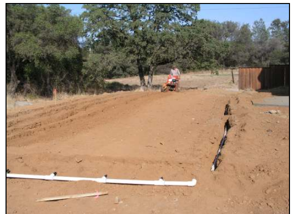
Installation of dripfield – drip lines are buried 6-10" below grade
