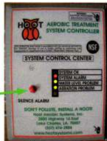
controller displaying alarm lights
