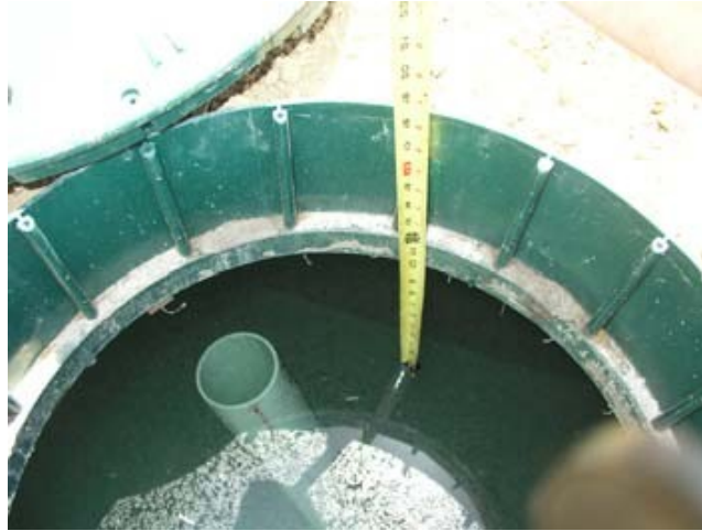
Begin filling the tank with water through the center chamber
