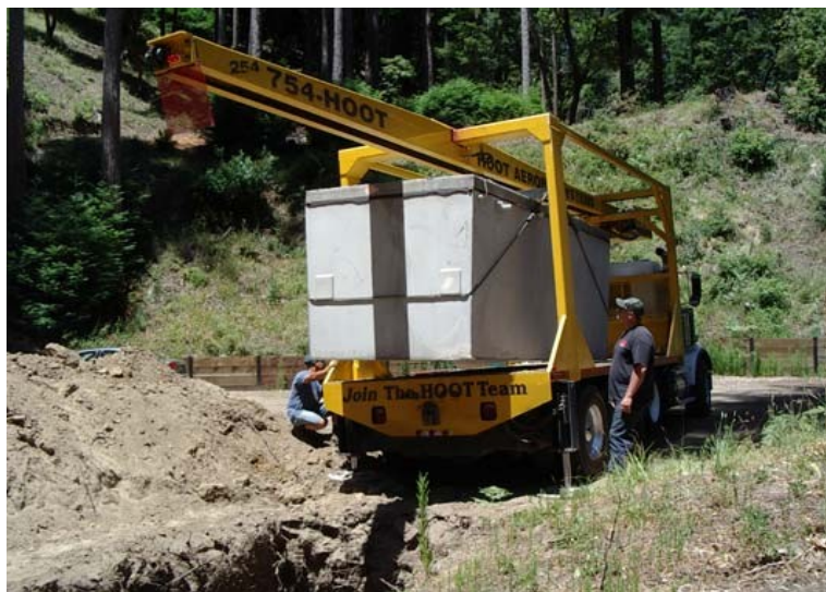
Delivery truck with mounted crane positioned for tank placement
