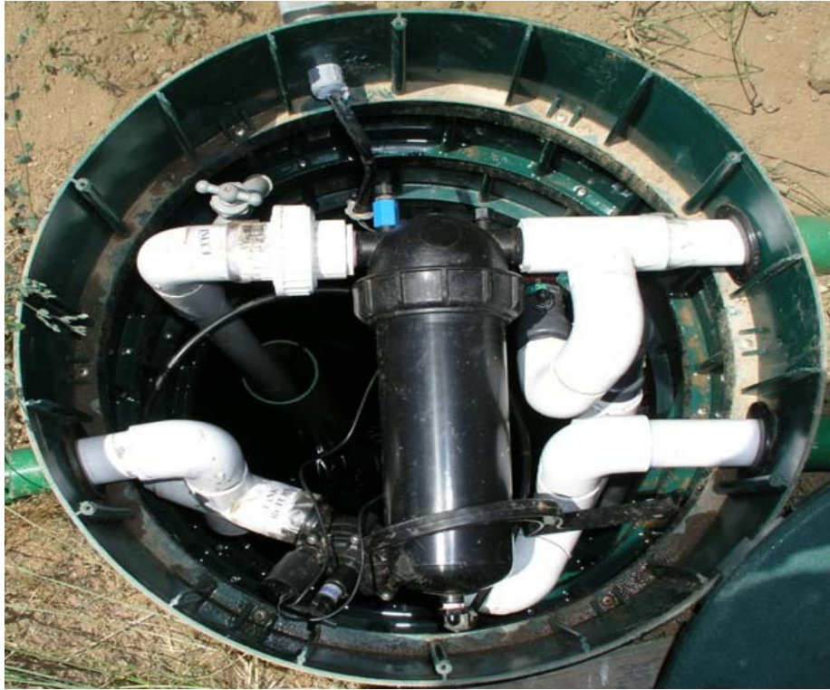
Typical Hoot tank-top connection layout — performed by SOS during commissioning
