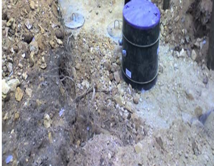
Risers brought to final grade with proper above-grade clearance
