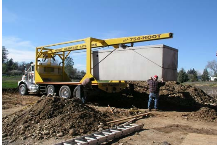
Tank inspection prior to placement in hole
