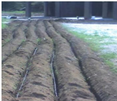
Typical dispersal field installation methods — trenching, plowing, prep, seeding, and grass establishment
