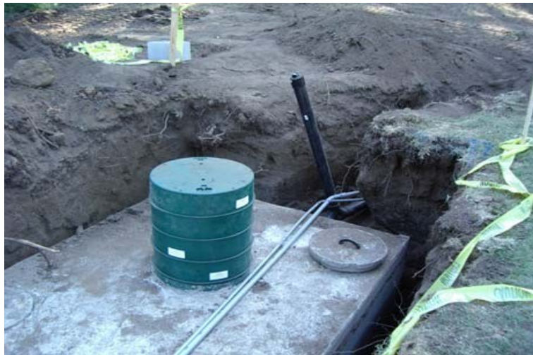
Tank set with sewer line connection and cleanout
